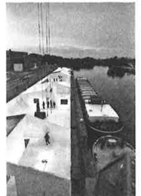
1 Sarah Melsens and Roberta Gigante, Use Me , conversion of gravel containers into an open-air venue for cultural activities, with the opening exhibition-cum-intervention, 'Grindbakken', by Rotor, Ghent 2012. Photo: Rotor.
