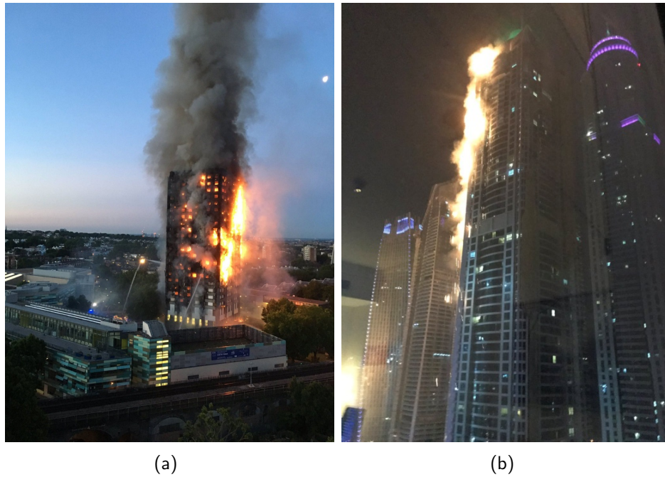
Figure 1.2: (a) London Grenfell Tower fire in 2017, (b) Second Torch Tower fire in 2017.
